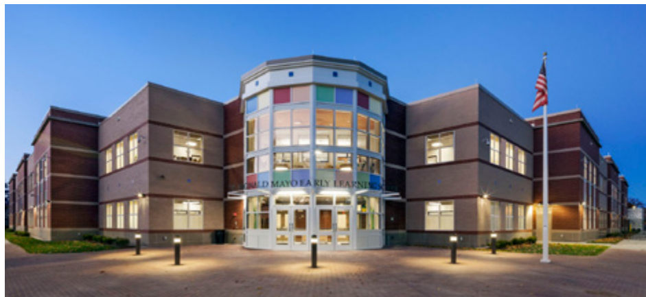
Main Entrance / all photos by Woodruff/Brown Architectural Photography
